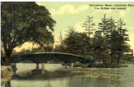
12 foot wide Foot Bridge to Island in Salisbury Pond
